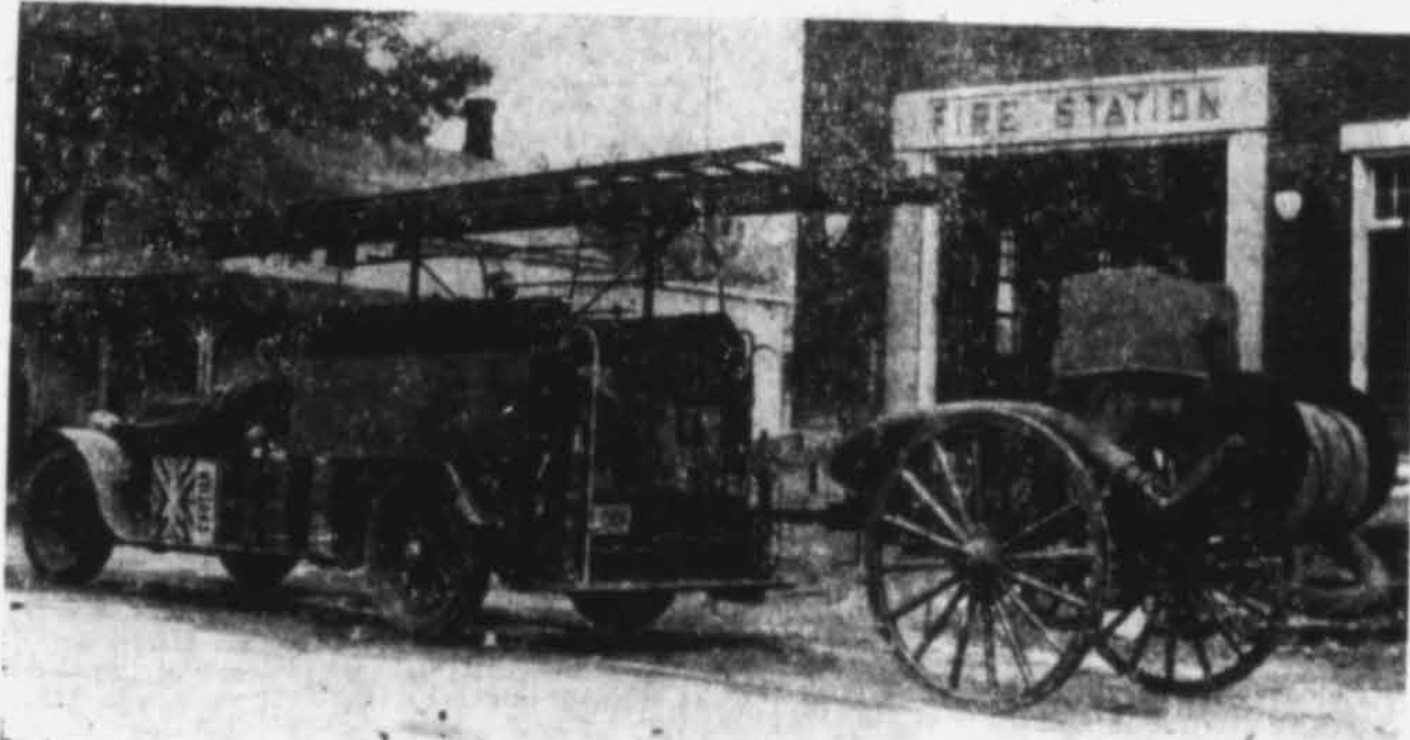
Above is shown some of the older type of fire fighting equipment which was used to combat fires in the Town of Huntingdon, outside of the present Fire Hall. The fire truck shown was used principally to carry the hose and equipment to a fire, it had no tank or pumper. At the rear is a pumper which was used when extra water was needed from the river or other available supply. It has served its purpose and has been replaced with more up-to-date and modern equipment.
