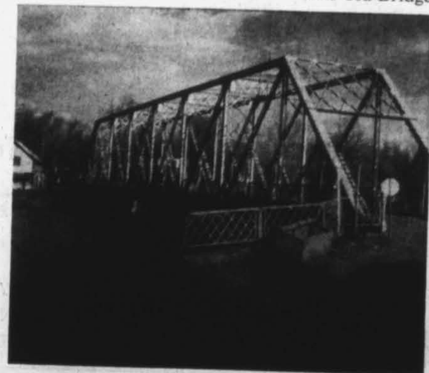
The Old Bridge
