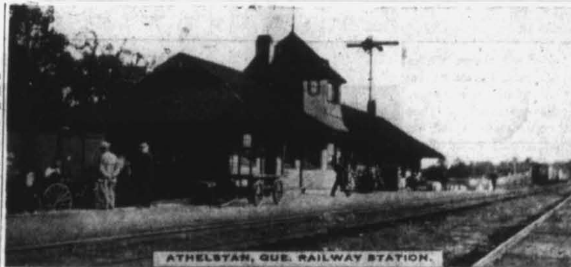
ATHELSTAN, QUE. RAILWAY STATION.
