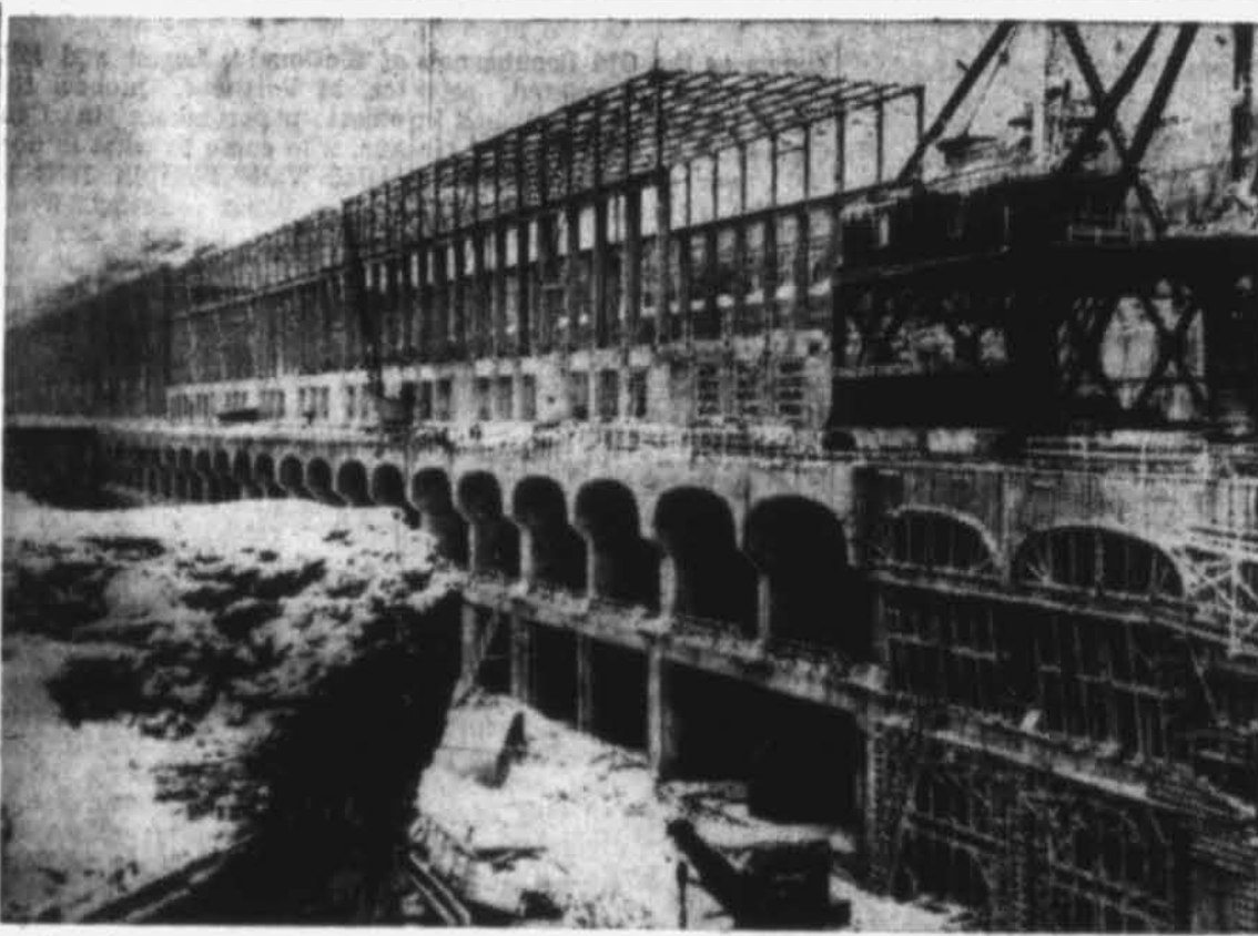
Beauharnois second phase takes shape. Beauharnois 1 at the left of the structure was in full operation when this photograph was taken.
